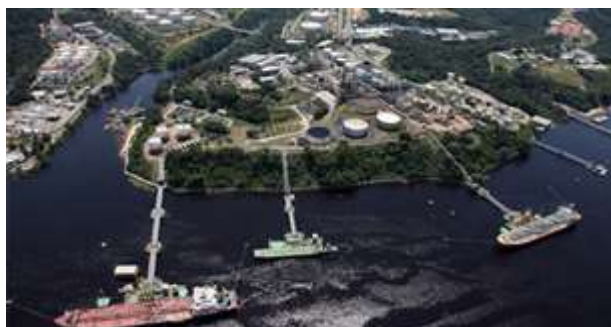
Source: REMAN – Refinaria Isaac Sabbá, Petrobras, 2020.
